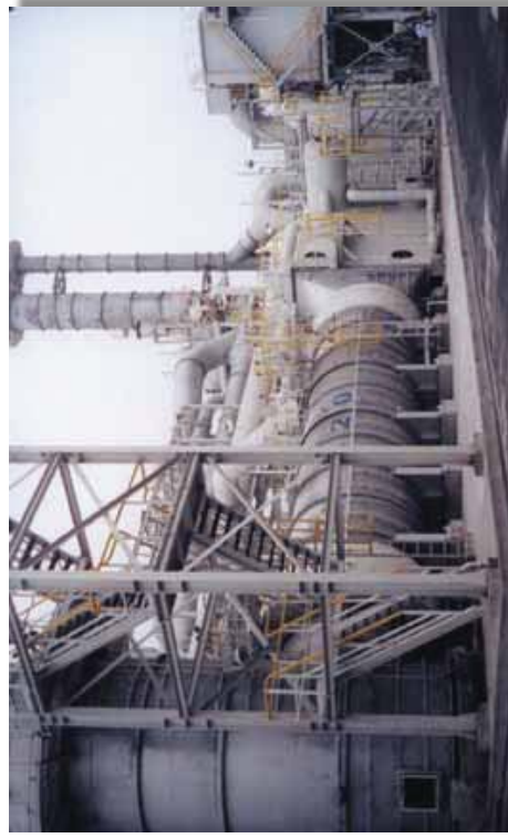
Liquid Waste Incinerator with SCR, Waste Heat Boiler and Baghouse. System Design Capacity = 129 MM Btu/hr
