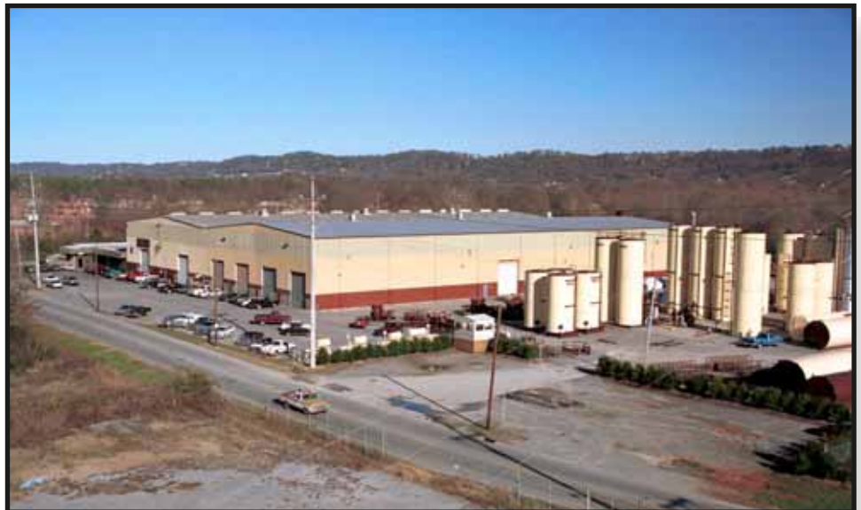
Heatec manufacturing facility and office in Chattanooga, Tennessee
